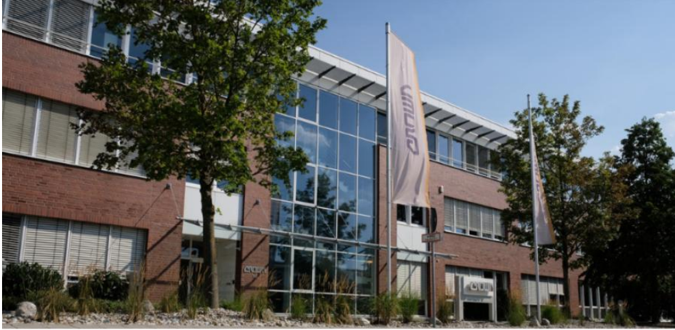
Crown EMEA headquarters in Feldkirchen, Germany.
